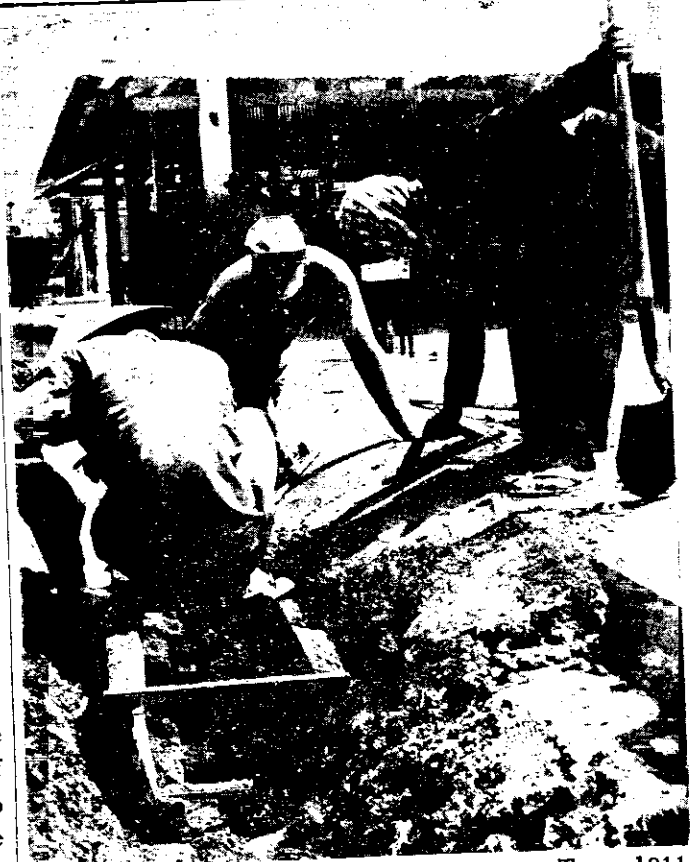
MARKET PLACE—A member of Seabee Team 1011 works with two Vietnamese workers, pouring and framing the gutter at the An Duc Market place.
